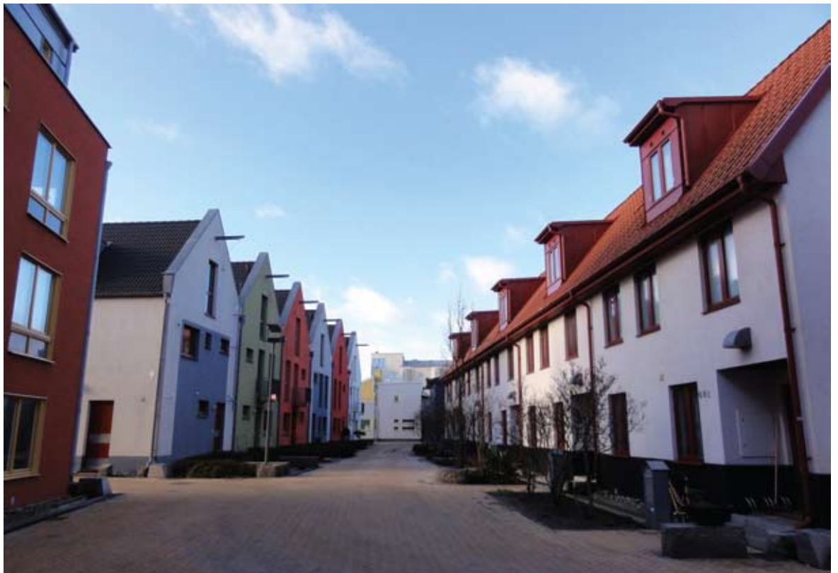
Street scene from Western Harbour, reminiscent of the Homezone approach adopted by Tenants First
