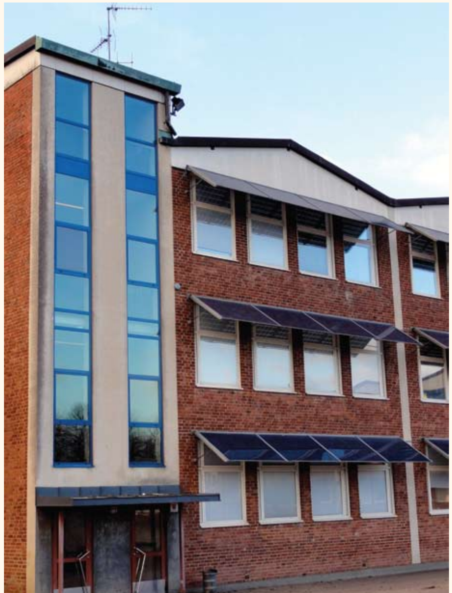
A school in Malmo using photovoltaic panels both to provide shading from the sun and generate power from the sun. Now that's clever!
