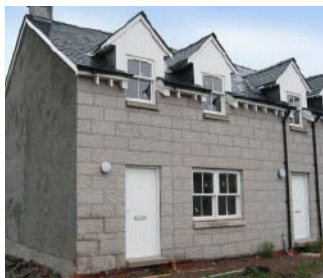
Three bedroom terraced houses
